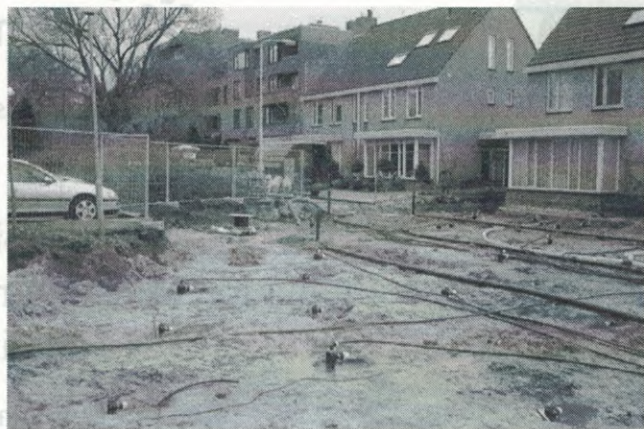
Fig. 1. Installing the electro-bioremediation system.
